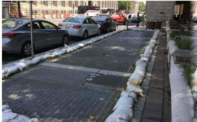
FIGURE 31. SANDBAGS BLOCKING STORMWATER FLOW FROM WASHINGTON METRO SUBWAY AIR VENT. SOURCE: G. GALLOWAY, UMD.
